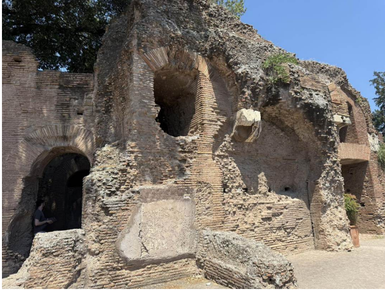
The brick-and-concrete chambers of the imperial palace (the Domus), built into the hilltop.
