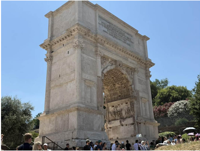
The single-bay arch on the Via Sacra; the inscription on this face is the 1821 restoration text, the ancient dedication being on the far side.
