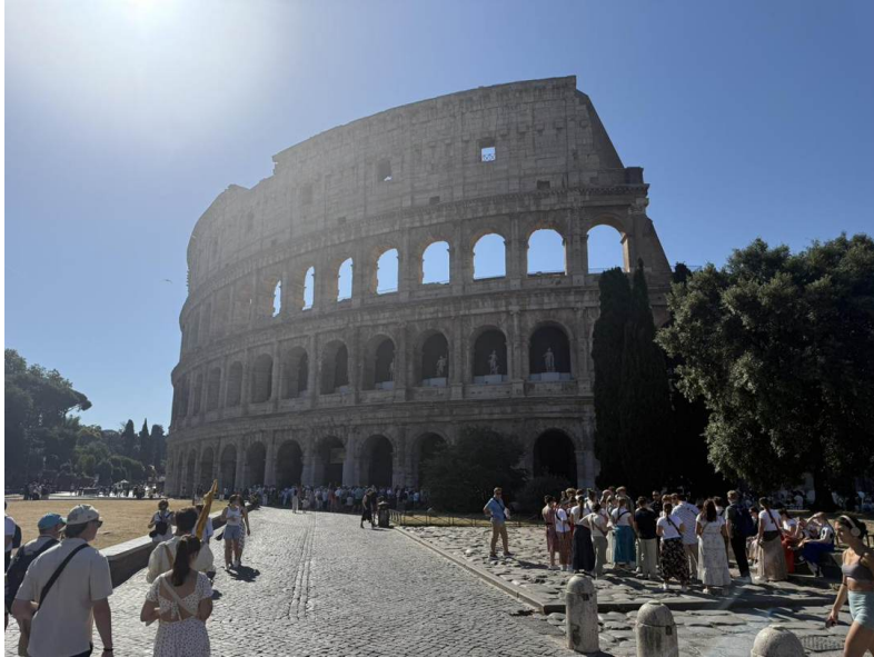
The great elliptical facade — three tiers of arches in superimposed orders, with the attic storey above.
