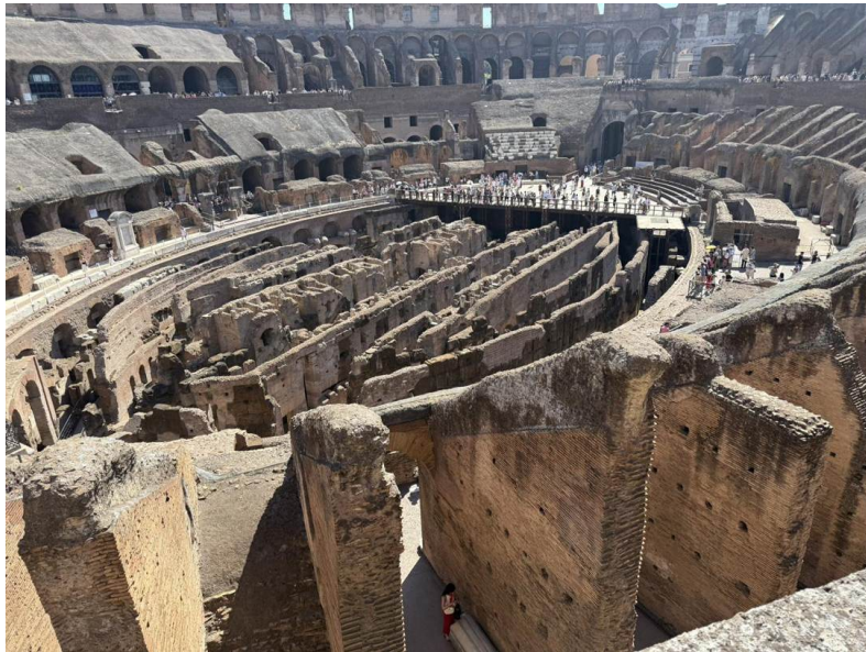
The vast interior — the cavea, the partly reconstructed wooden arena floor, and the exposed underground works.
