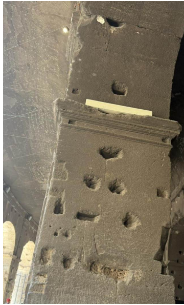
A travertine pier riddled with holes — the sockets of iron clamps that were later prised out.
