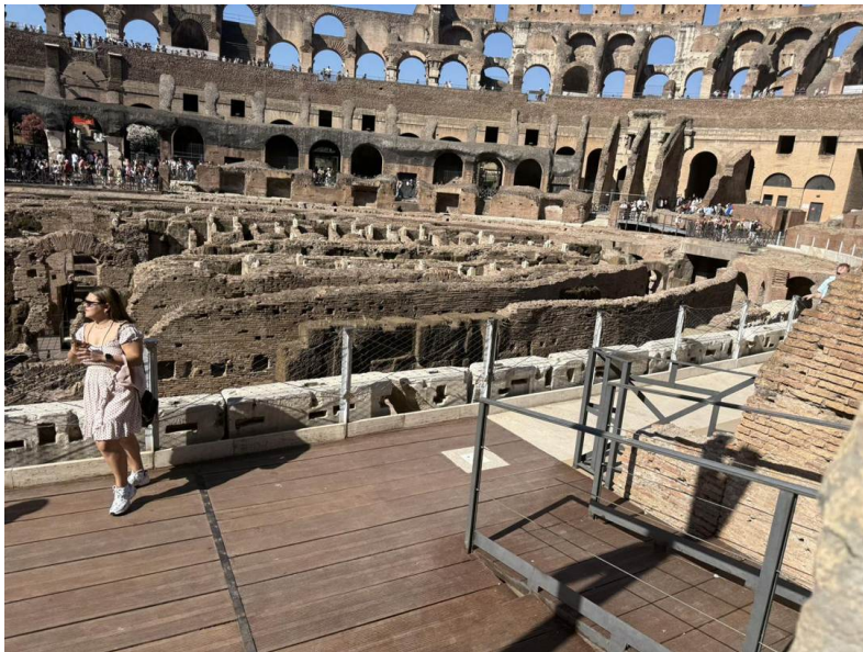
Part of the wooden arena floor, rebuilt over the hypogeum it once concealed.
