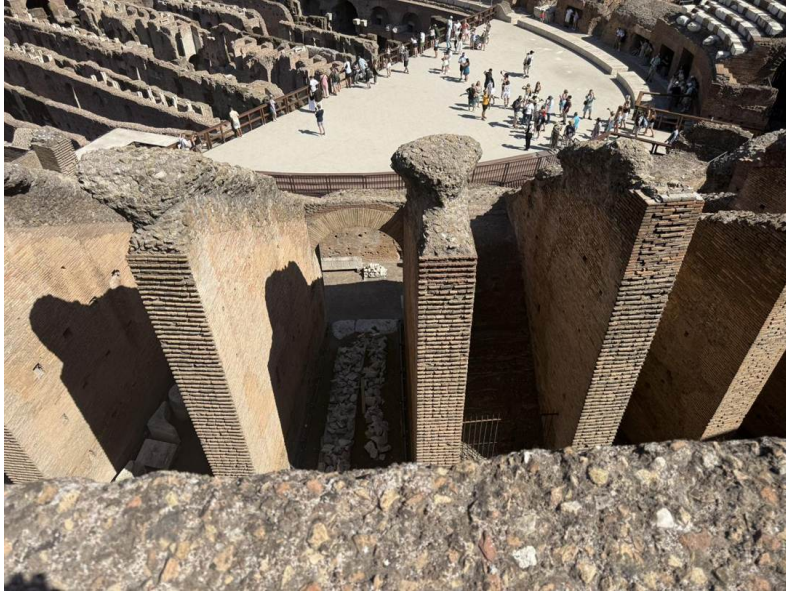
Looking down into the hypogeum: the brick piers and channels that ran beneath the arena floor.
